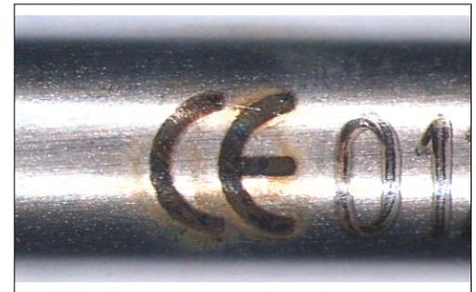
Slight corrosion at the laser engraving
